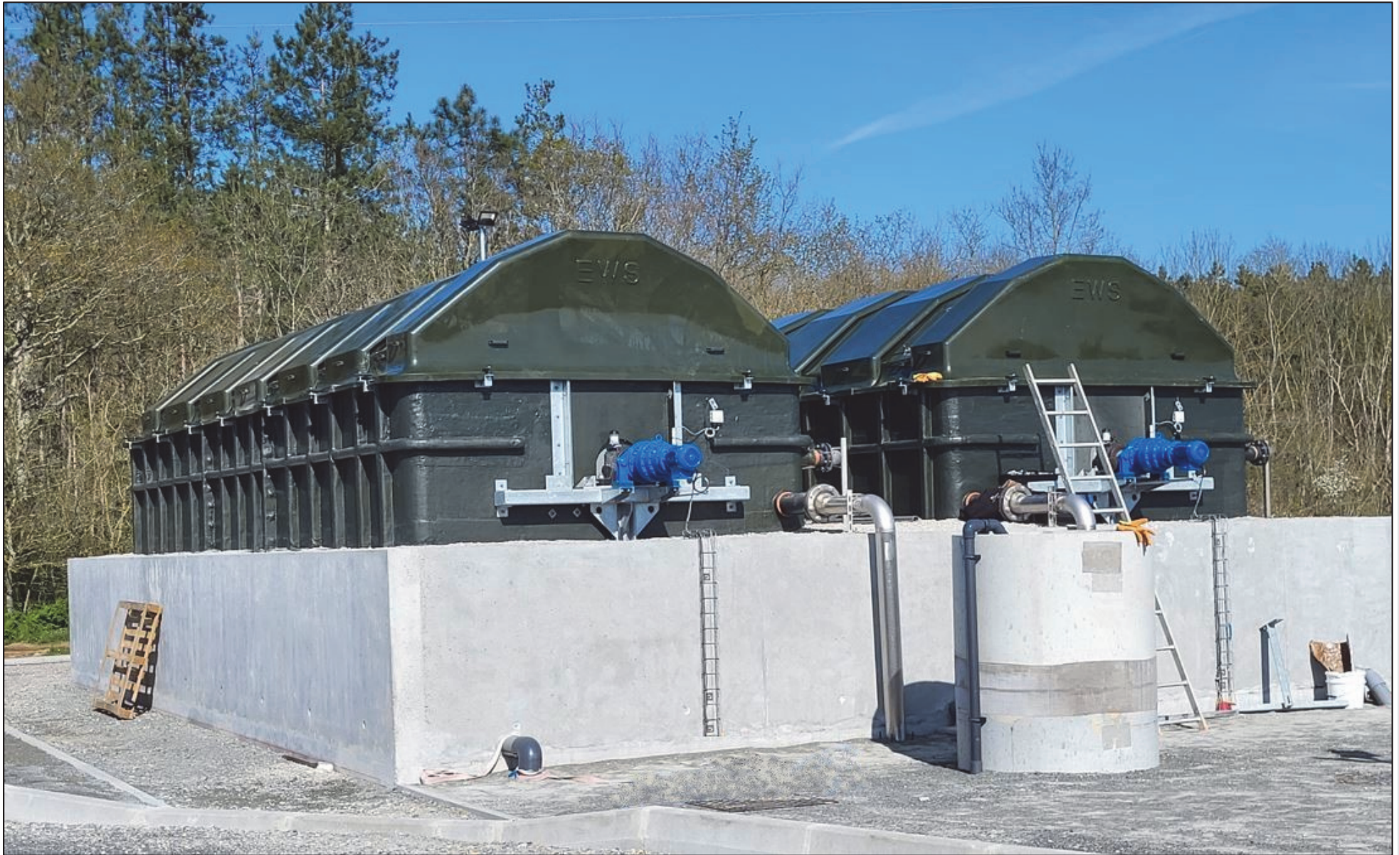
800 PE WwTP – Two EWwS NiFAS® RBC units installed above ground
